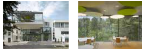
Office building Glatten, DE Ref. 1277* Photo: Roland Halbe
