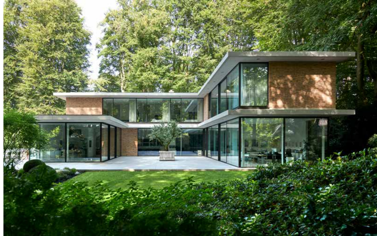
cero III Villa Hamburg, DE Architect: Meyer Terhorst Architekten Photos: Christiane Koch Ref. 789*
