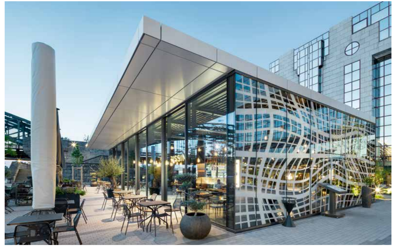
cero III Restaurant Grissini Cologne, DE Architect: Gatermann + Schossig Photos: Constantin Meyer Ref. 1585*
